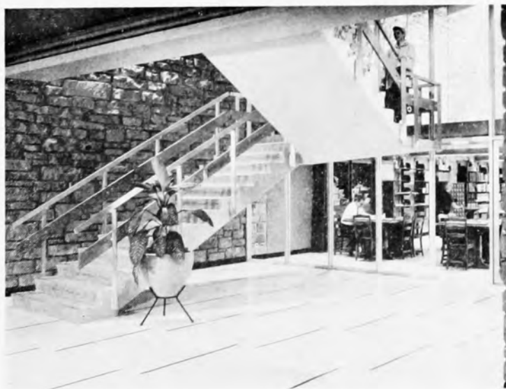
The Lobby in the Administration Building
